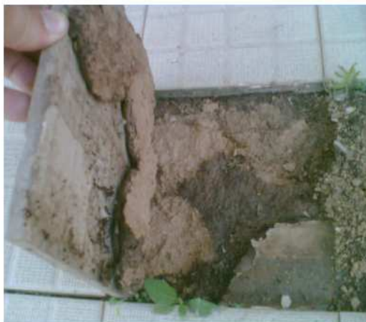
Installation using the thick-bed technique + water
