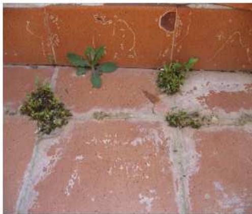
Deteriorated joints
